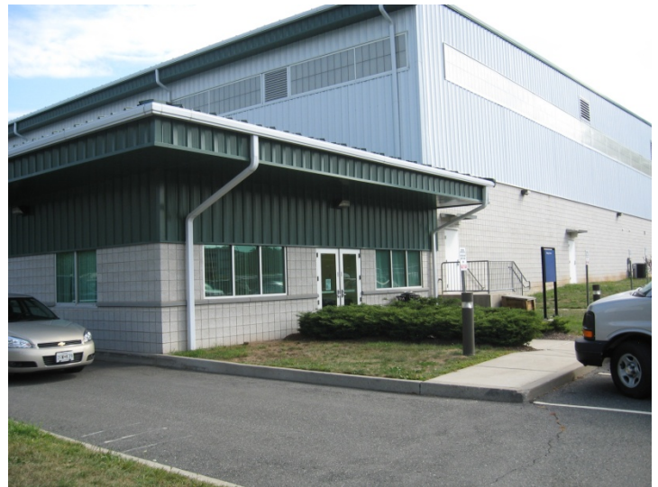
Parking Services Entrance
